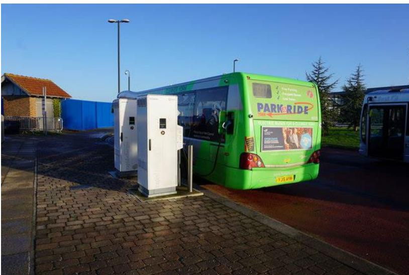
Figure 22. Curbside Charger with Electric Bus
