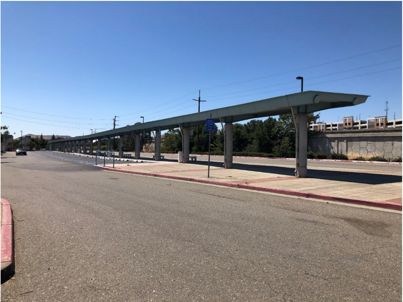
Figure 36. South side of the Pleasanton-side Bus Island and ADA Parking
